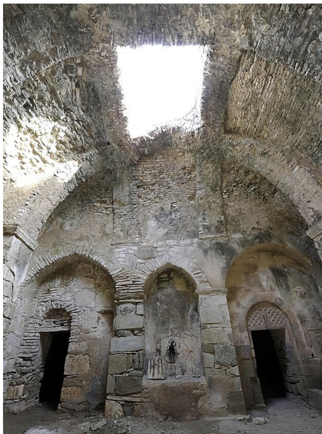
Fig. 3.12. Bëri Elts'i, Arts'akh (13th century). The common narthex ( gawit' ) of two chapels. Internal view towards the east. Vault with pairs of crossed arches. Photo: H.H. Khatcherian
