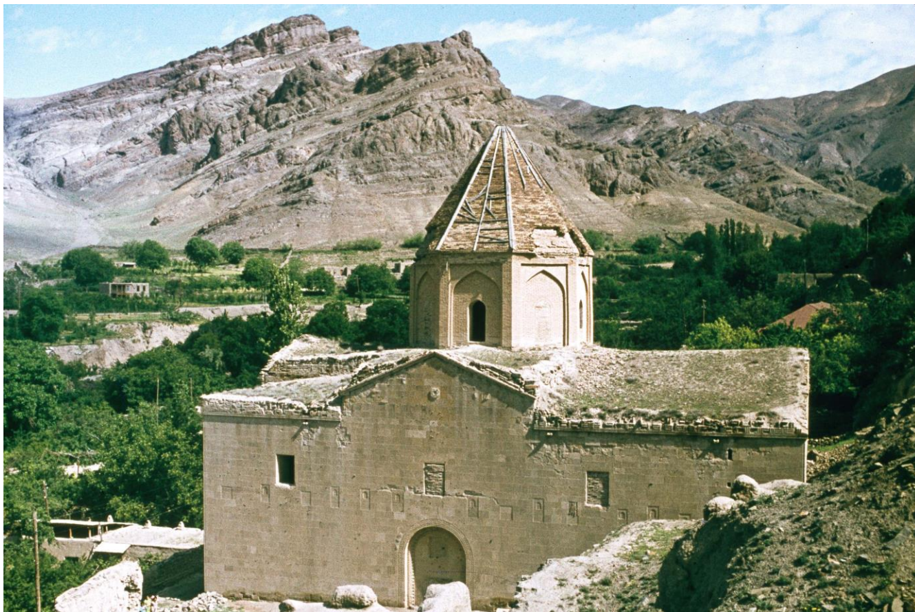
Fig. 4.6. Church of Surb K'ristap'or (1671–1675), Agulis, region of Nakhichevan. South view. Photo: A. Ayvazyan (1980s), UIOTC v-21843_01, Argam Ayvazyan's Fund
