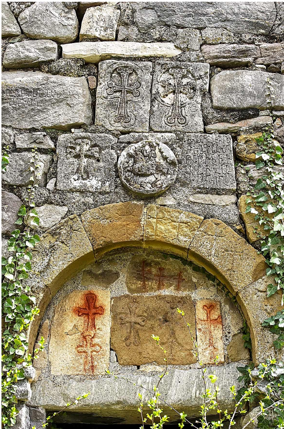
Figure 5.39. Monastery of Surb Elisha (13th century), Arts'akh. The chapel south of the main church. Detail of the west façade above the door. Photo: H.H. Khatcherian
