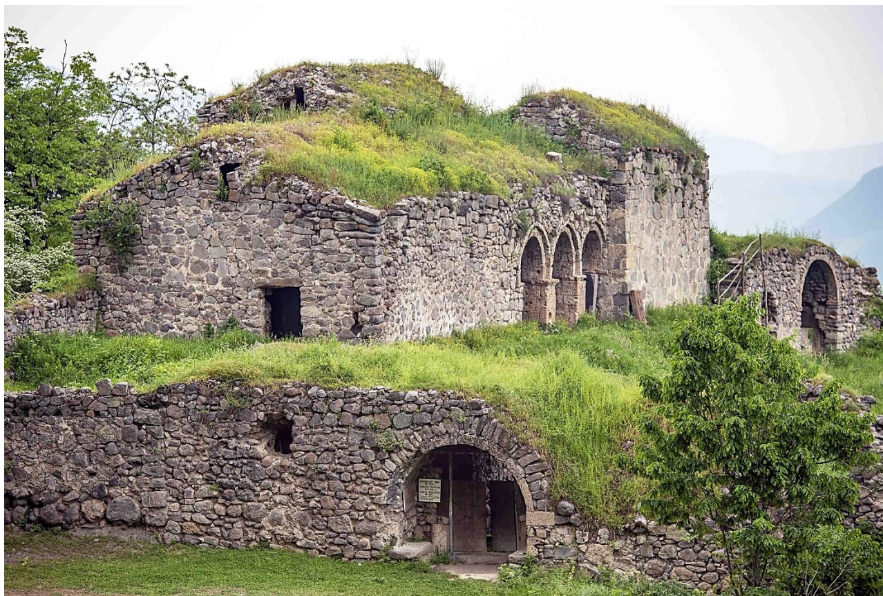
Figure 5.57. Monastery of Surb Yakob (13th century, 1691), Arts'akh. View from the southwest towards the ecclesial complex. Photo: H.H. Khatcherian
