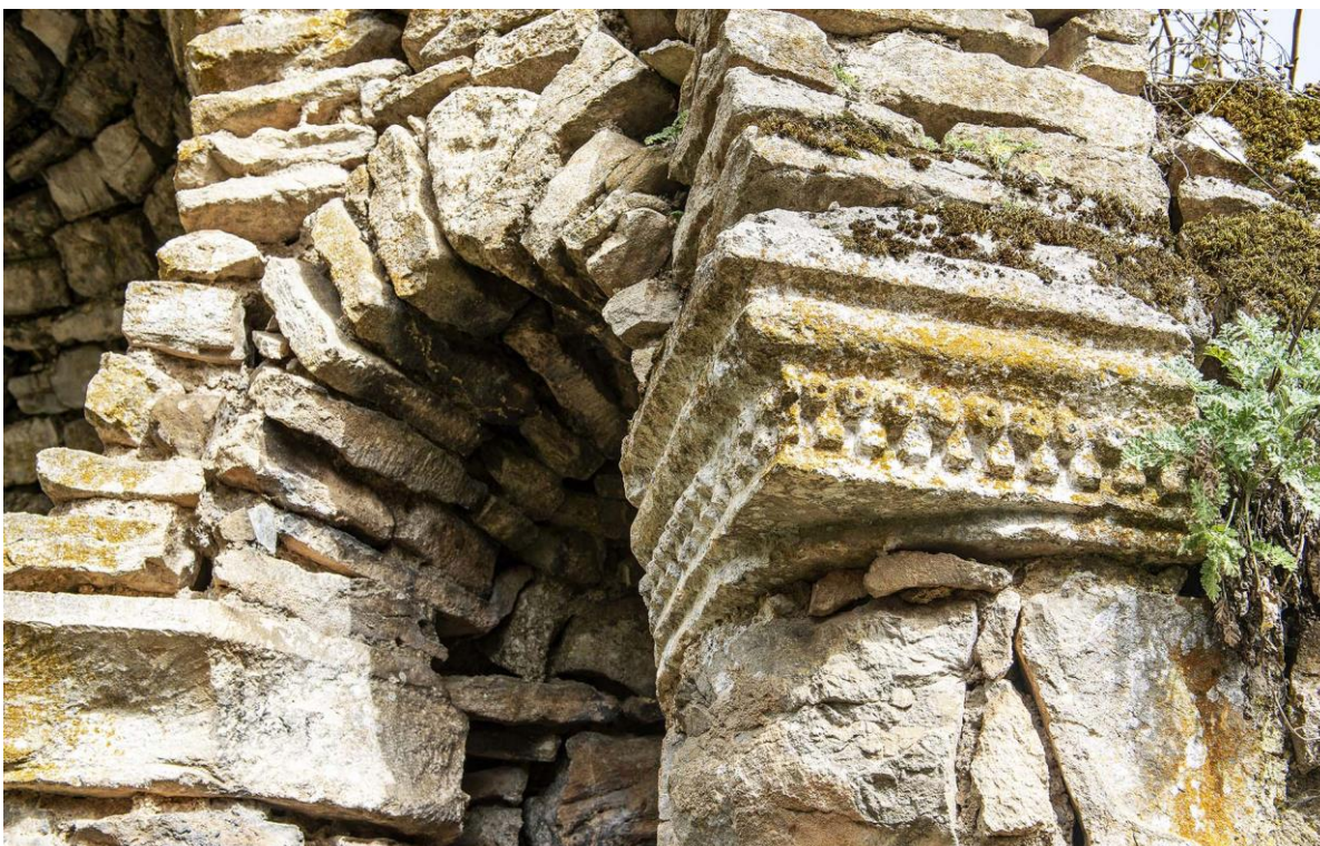
Figure 5.36. Church of Ökhtě Děrni, Mokhrenis (ca 6th–7th century), Arts‘akh. Impost of the northern corner of the apse. Photo: H.H. Khatcherian
