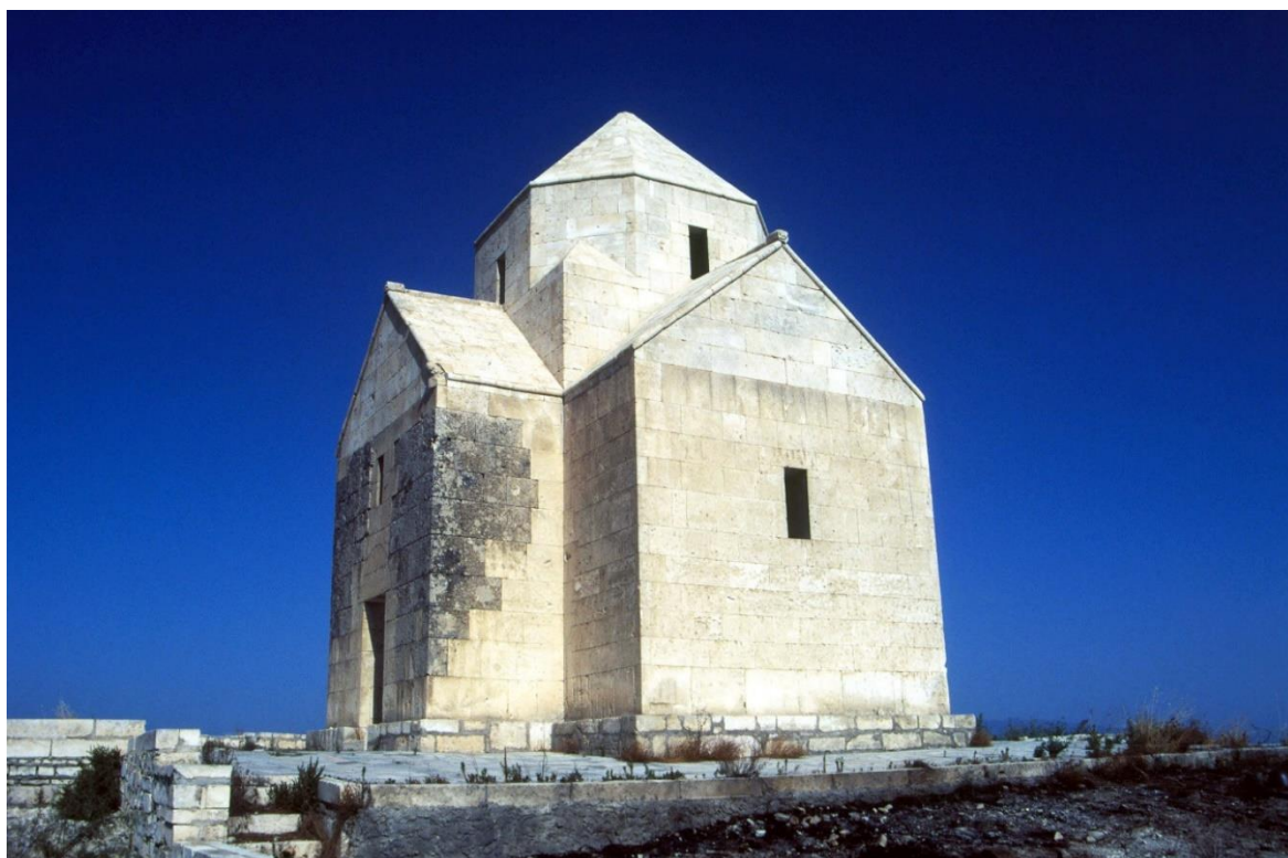
Figure 5.16. Vank‘asar, chapel (probably, 7th c.), Arts‘akh, rebuilt by Azerbaijani authorities in the middle of the 1980s. View from the southwest.
