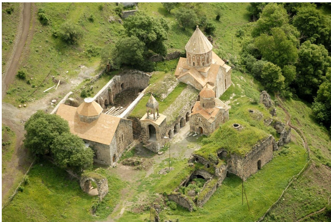
Figure 5.10. Dadivank´ monastery (late 12th–13th century), without the southwestern residential group, Arts´akh. Aerial view from the southwest. Photo: H.H. Khatcherian
