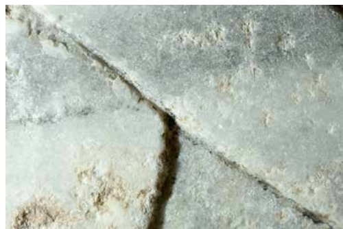
Fig. 6. Detail of the lintel showing a straight line carved with a chisel; note the V-shaped profile of the line.
