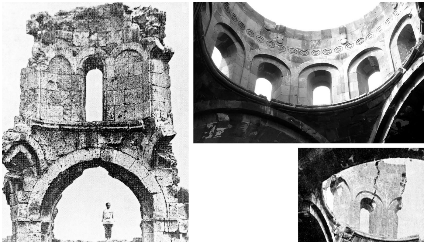
Fig. 7. Row of flat, arched niches inside drums of 7th-century Armenian churches: Fig. 7a. Aygeshat (ca. 630–40). Photo: Archives of the Museum of History of Armenia (Yerevan)
