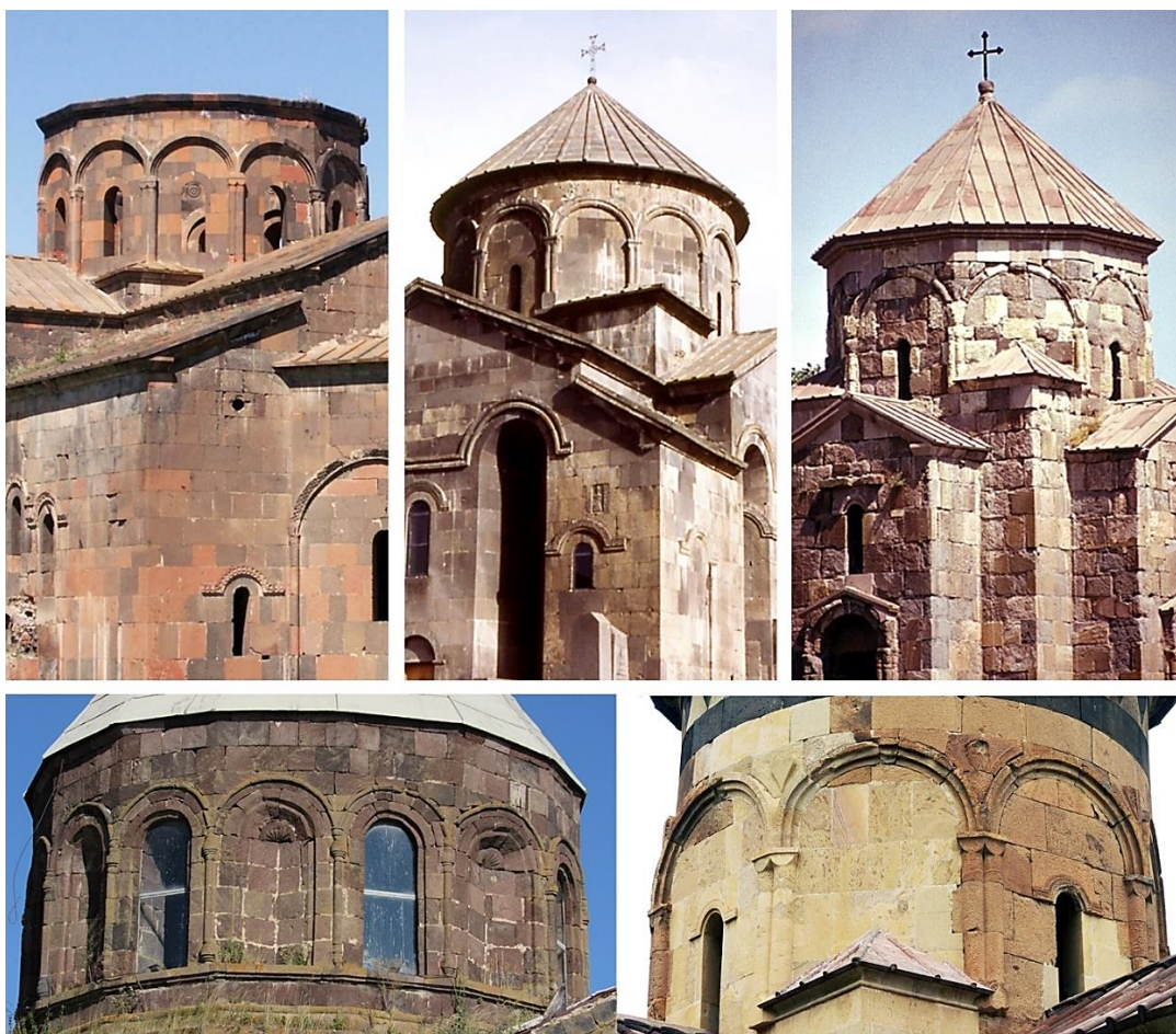
Fig. 10. Blind colonnade-arcade on the drums (outer face) of Armenian churches of the second half of 7th century: Talin (rebuilt), Sisian, Voskepar, Dədmashen (rebuilt), Hnevank. Photos: Patrick Donabédian
