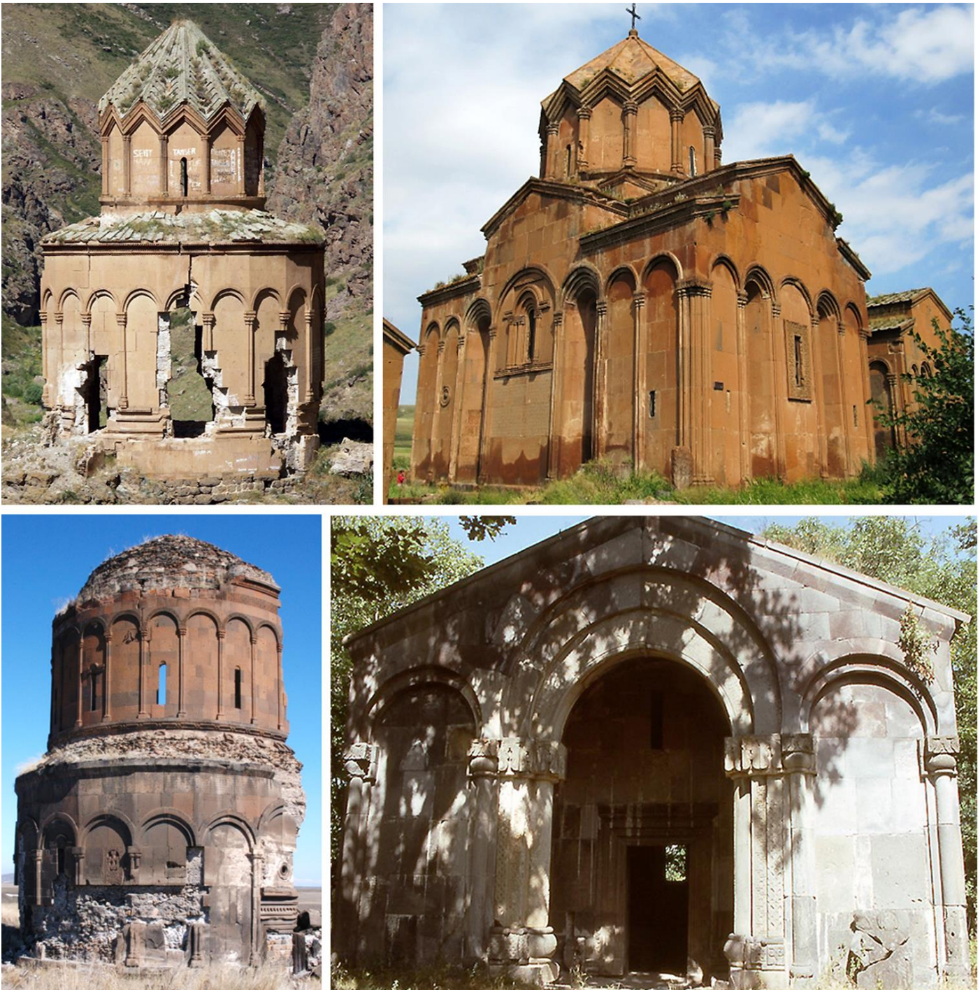
Fig. 17. Slightly recessed “niches” under the arches of some 11th-century Armenian churches: Khətzkonk, Saint Sergius (1024), Marmashen (1029), Ani, Saint Savior (1036); more marked at Noravank of Bghen (1062). Photos: Patrick Donabédian
