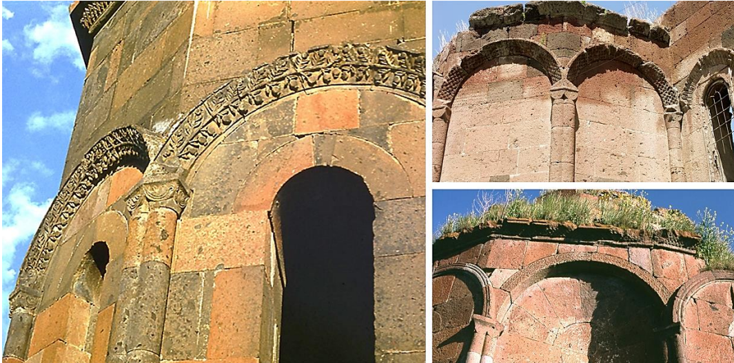
Fig. 9. Blind colonnade-arcade on the apse and conches of Armenian churches of the second half of 7th century: Talin, Artik, Irind. Photos: Patrick Donabédian
