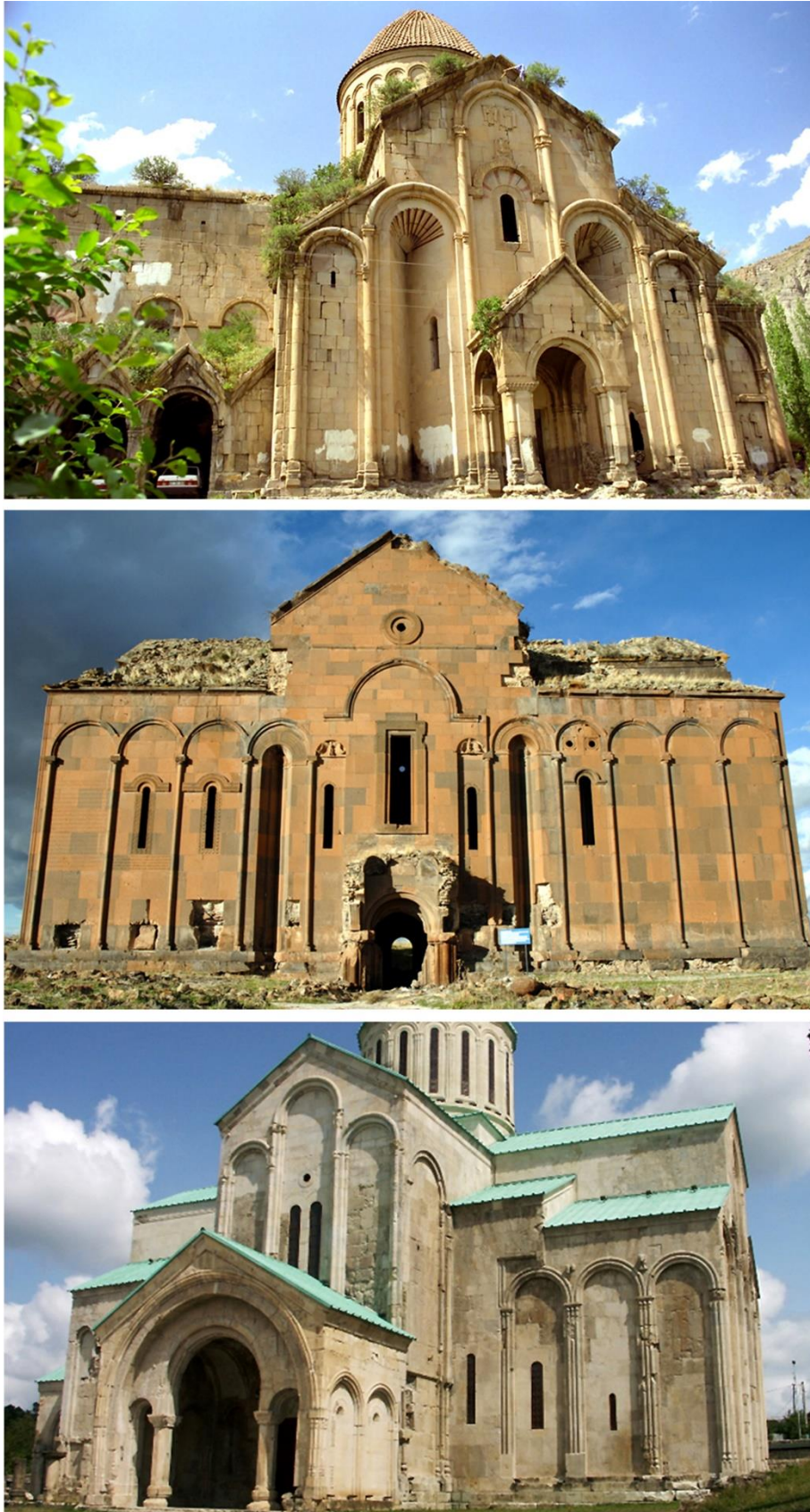
Fig. 16. Single-shaft colonnade on the three major cathedrals of the region: Oshk'(i) (T'ao/Tayk, 963-973), Ani (989-1001), Kutaisi (1003). Photos: Patrick Donabédian
