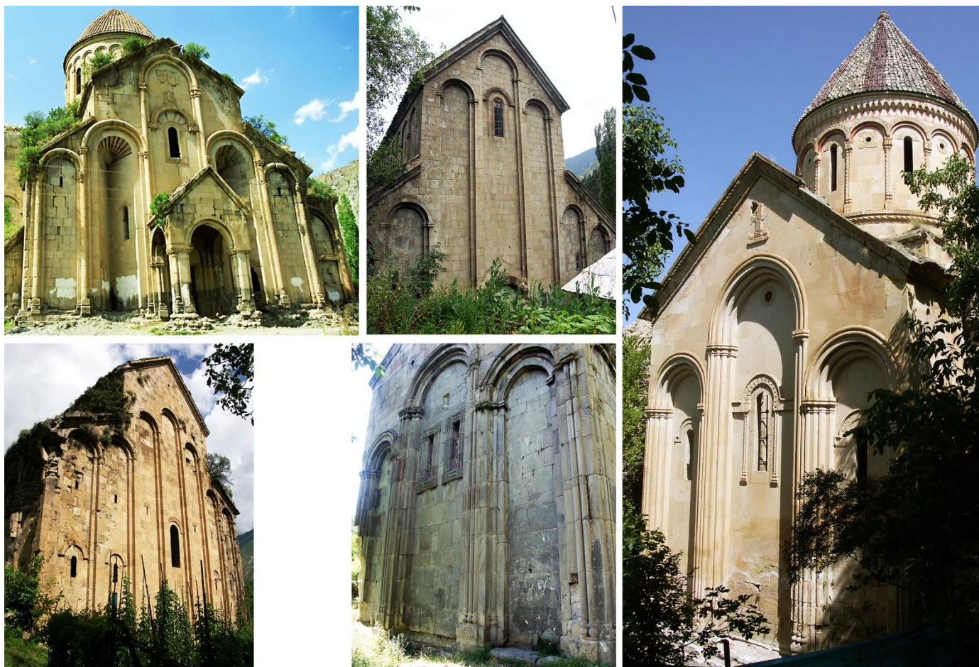
Fig. 18. Progressively increasing height of the arcades on churches of Tayk/T'ao in the 10th-11th centuries: Oshk'(i) (963-973), Parkhar/Parkhali (970s), Chordvan(k)/Otkhta Ek'lesia (970s), T'beti (early 11th century), Ishkhan(i) (1032). Photos: Patrick Donabédian
