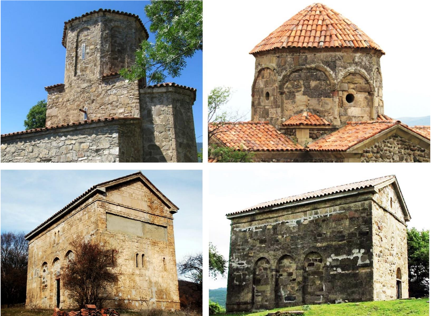
Fig. 12. First rows of flat, arched niches and first blind arcade in Georgia during the “transitional” period (ca. 8-9th centuries).
