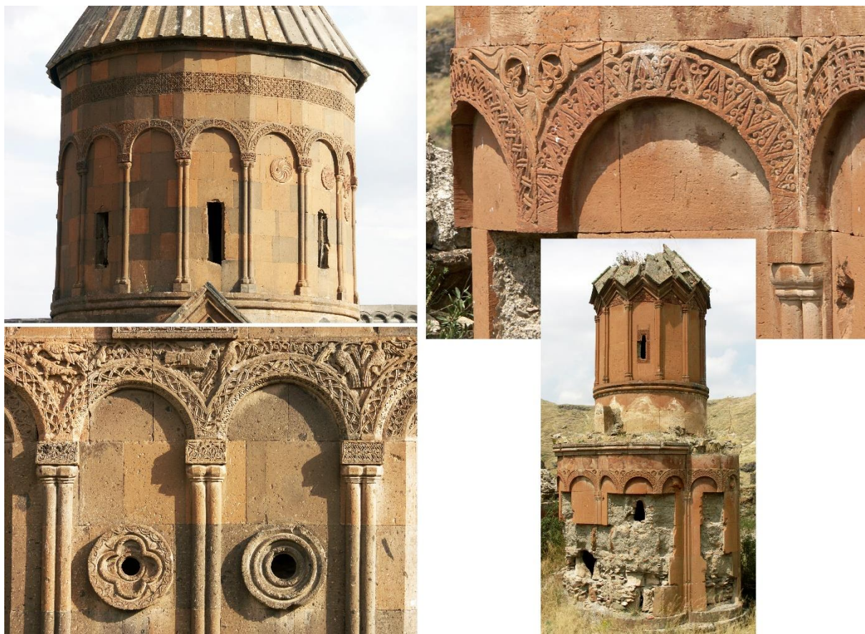
Fig. 19. Blind arcade on Armenian churches of the early 13th century in Ani. Right: chapel of the Convent of the Virgins (before 1215); left: church of Saint Gregory the Illuminator of Tigran Honents (1215). Photos: Patrick Donabédian
