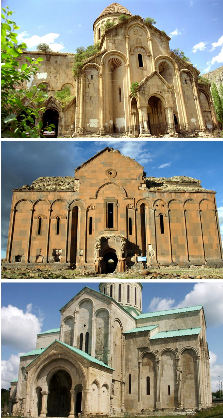
Fig. 16. Single-shaft colonnade on the three major cathedrals of the region: Oshk'(i) (T'ao/Tayk, 963-973), Ani (989-1001), Kutaisi (1003). Photos: Patrick Donabédian
