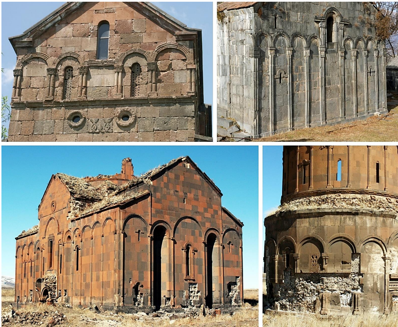
Fig. 15. Blind arcades on Armenian façades of the 10th-11th centuries: Byurakan, Saint John (early 10th century), Sanahin, Saint Savior (966-972), Ani, cathedral (989-1001), Ani, Saint Savior (1036). Photos: Patrick Donabédian
