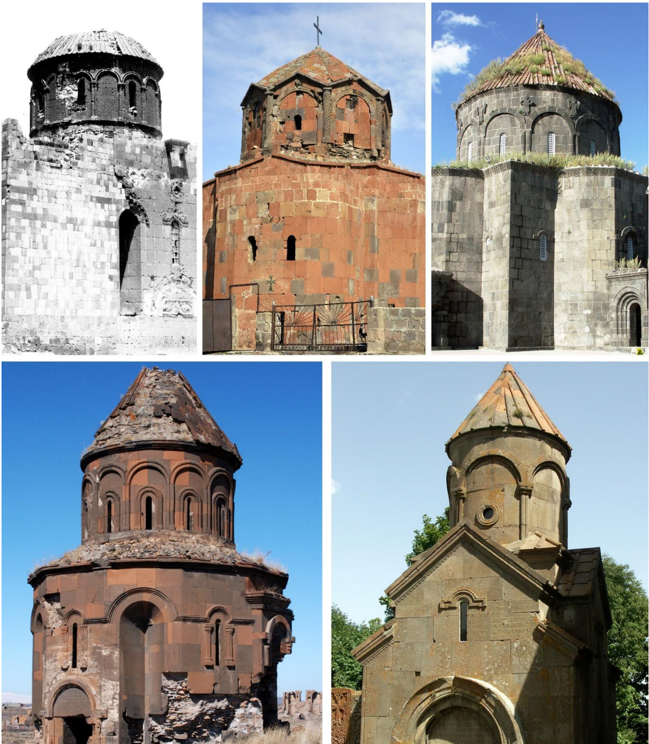
Fig. 14. Blind arcades on Armenian drums of the late 9th-11th centuries: Oğuzlu (890s, restored in 1001), Zarinja (late 9th-early 10th century), Kars (930s), Ani, Saint Gregory of the Pahlavunis (late 10th century), Kecharis, Holy Sign chapel (1051). Photos: Patrick Donabédian; except Oğuzlu: Archives of the Museum of History of Armenia
