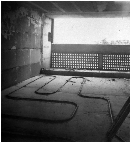
Figure 24. Apartment's coil (FLC L3-1-21c)
