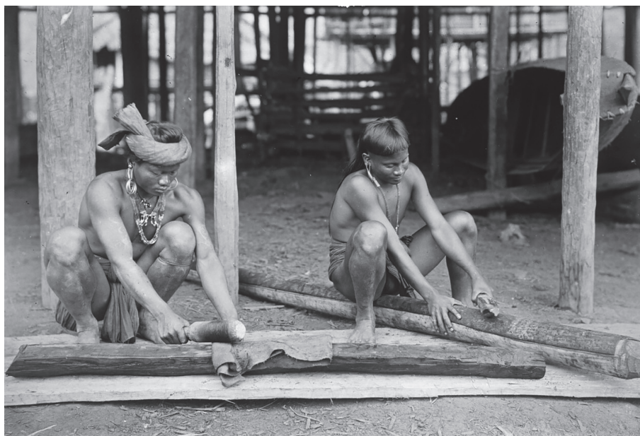
Fig. 11. Manufacturing bark cloth, Kayan, upper Mahakam
