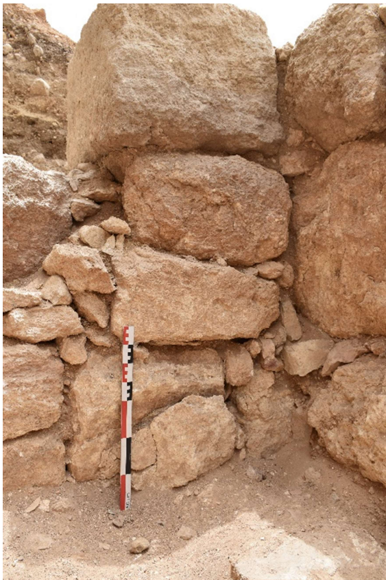
Fig. II13. Wall W1 on the right shows the shape of its construction with blocks of different modules and the use of smaller stones as filling. It also shows the connection between walls W01 and W60.
