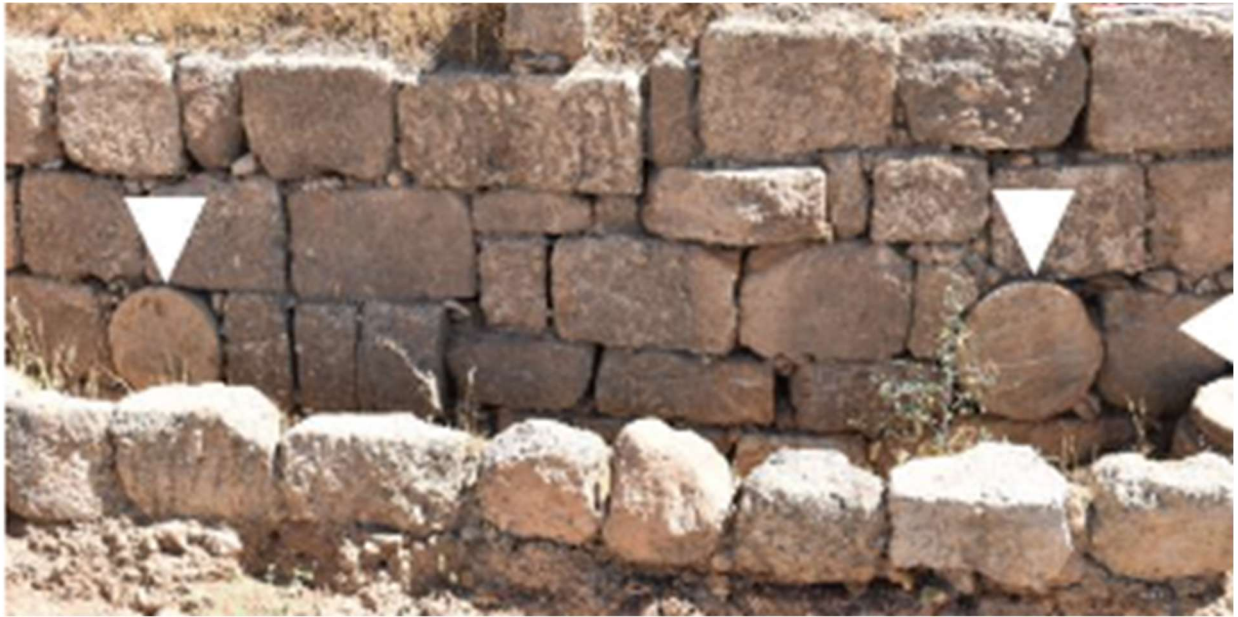
Fig. VIII.3. Drums used inside the masonry of wall W2.
