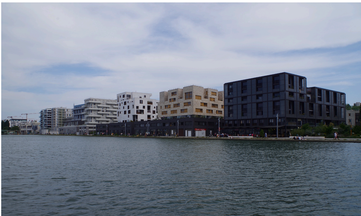
Fig. 9. Recent real estate developments along the Canal de l'Ourcq. Photo by Basile Michel, 2023.
