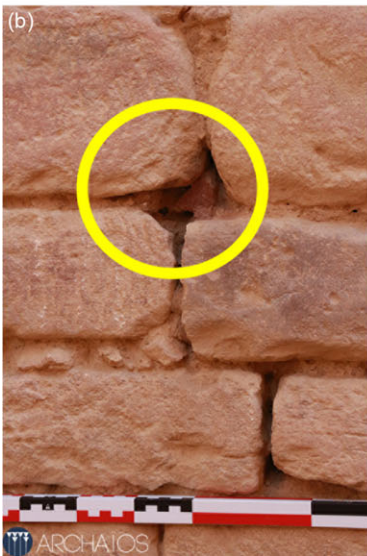
Figure 4. General view from west of the façade of the U54 with the sampling point of the mortar (in yellow) (picture by Piero Gilento, Archaiōs; b. Detail of the sampling point (picture by Giovanni Pesce, Northumbria University); c. Macrophotography of the charcoal sample embedded in the mortar (picture by Giovanni Pesce, Northumbria University).
