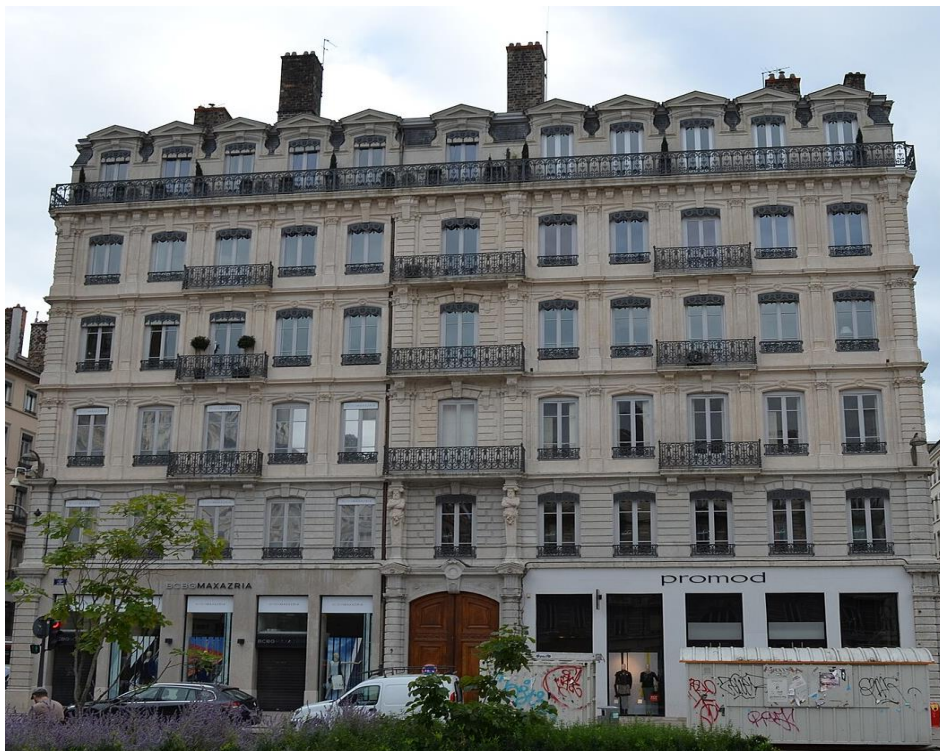
9, place des Jacobins (2 e arrondissement, cliché Farfounoux)
