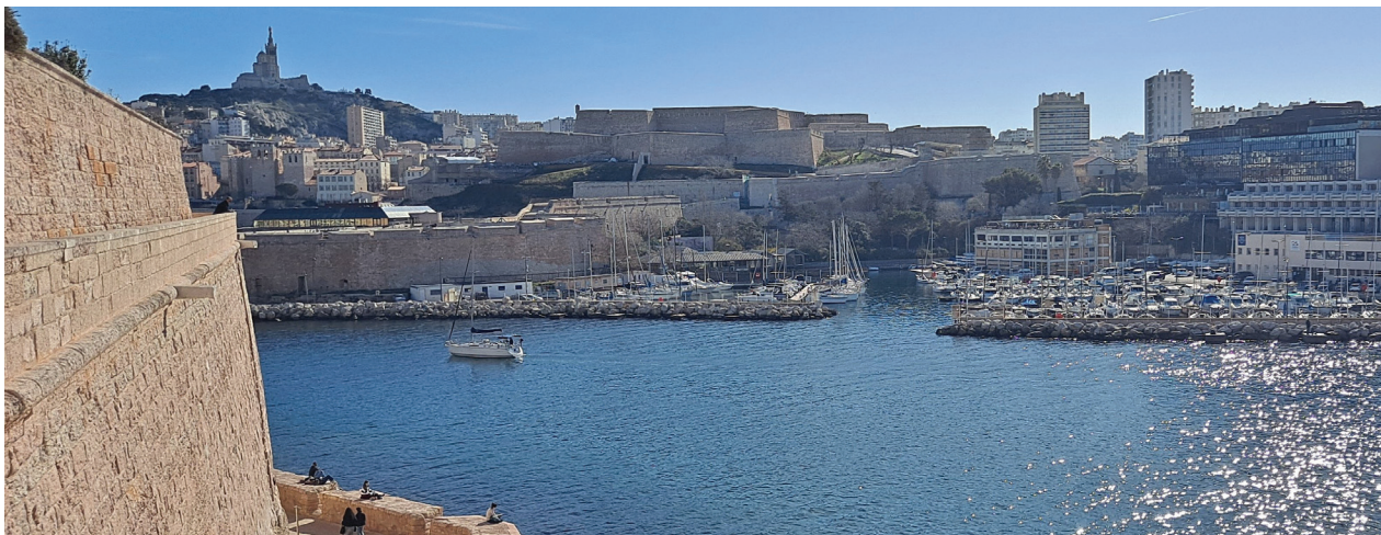
Fig. 2. The former Fort Saint-Nicolas as seen from Fort Saint-Jean located on the other side of the harbour. The fortification was divided in two by a boulevard and renamed Fort Ganteaume (lower fort) and Fort Entrecasteaux (higher fort) in 1887 (photo by J.Y. Blaise, 2024)
