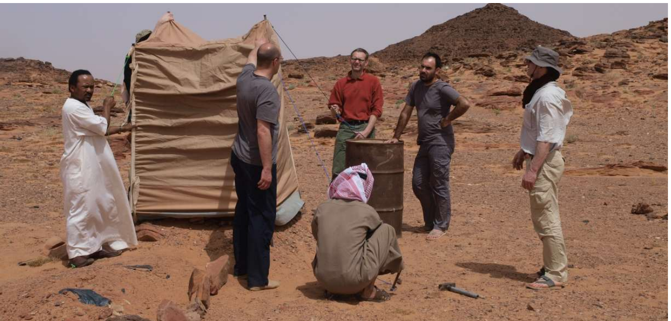
Fig. 23 : Installation of sanitary
