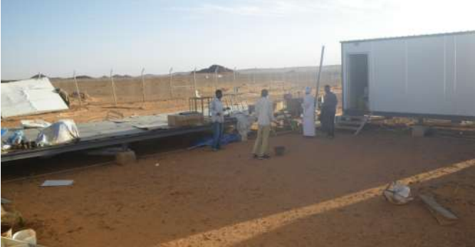
Fig. 28 : Prefabricated housing unit blowing out
