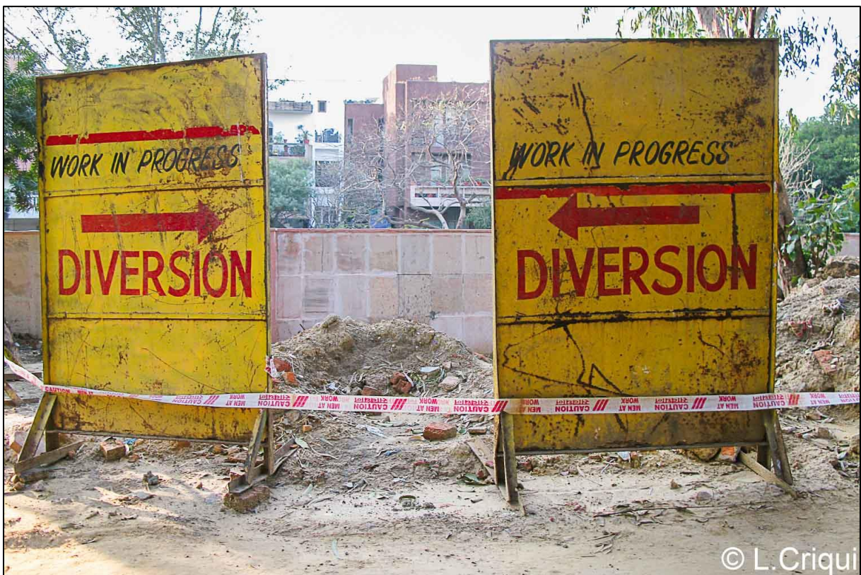
Photo 1/D. Work in progress (Delhi, 09/02/2013)
