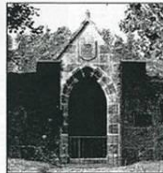
Newly restored arch of the mausoleum.
