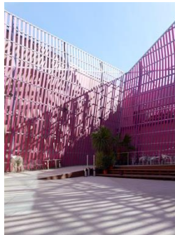
Figure 64, bâtiment SMAC, Nîmes
