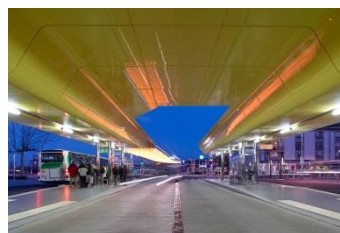
Figure 80, Gare multimodale, Saint-Nazaire, Tetrarc
