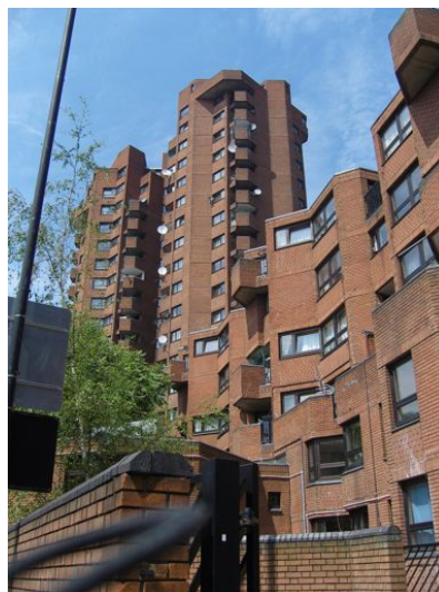
Photographie 20 : World's End Estate
