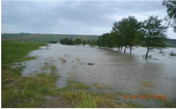
Fig. 6.57 Ezer Pond – dam’s body –flooded downstream bench
