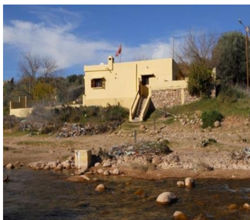
Photo 4.1 : Station de Taghzirt.
