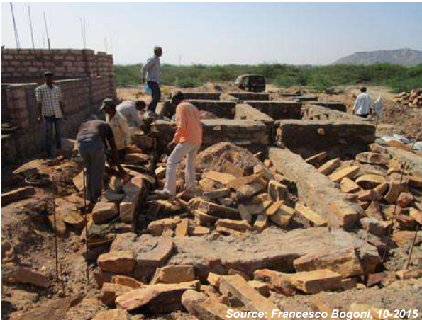
Image 34. Demolition of houses’ plinth because of improper execution (left). Image 35. Delays of installment release in a beneficiary’s checkbook (right).
