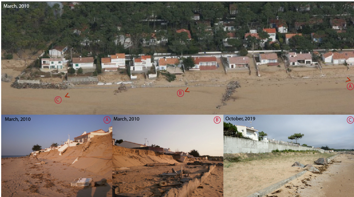
Figure 4 : The shoreline's retreat and damage on protection works in the aftermaths of Xynthia. La Tranche-sur-Mer – South of the Clémenceau beach.
