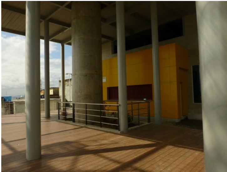
The pillars built for the teleferico
