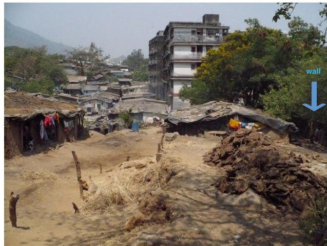
Figure 6.4. Four-storey building in Kailash Nagar constructed across the boundary of the SGNP. Semi-solid rented houses are on the left side, inside the park.
