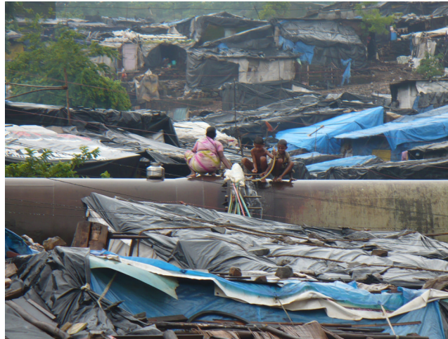
Figure 6.10. Boring a municipal water pipeline to get water access in Damu Nagar.
