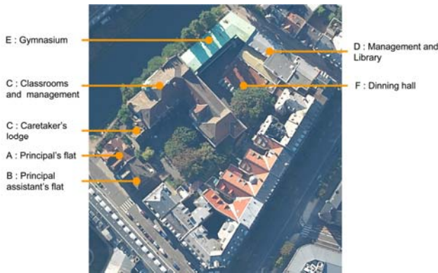
Fig. 1. Aerial view of "Pontonniers International High School" area in Strasbourg
