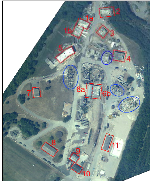
Figure 1: Aerial image of the test area (in red: undamaged buildings, pancake collapses, inclined planes; in blue: heaps of debris, outspread multi layer collapse)
