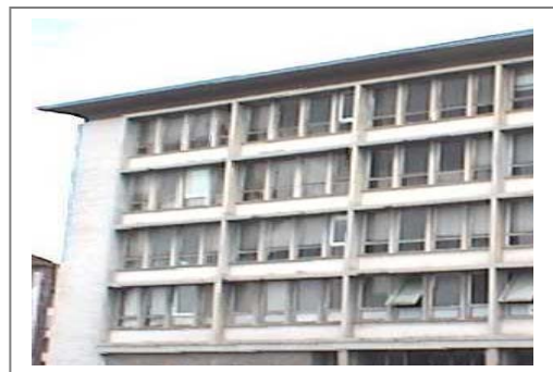
Figure 1. Photograph of the building under study
