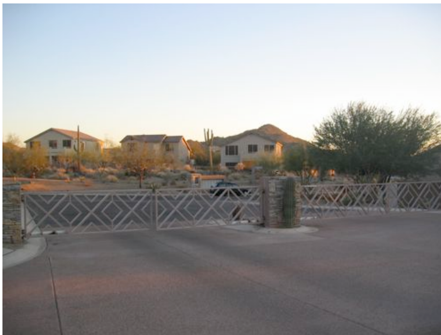
30 Figure 1 – A standard gated community near Pheonix (Arizona), secured by an automated gate. © Le Goix, 2007
