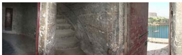
Figure 3: A view from the inside of the signal light tower, showing the spiral staircase and the balcony on level 3 (UMR MAP, 2006).
