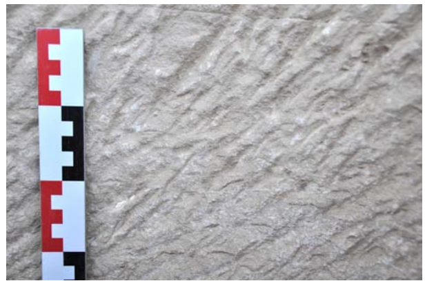
Fig. 66. Inside wall of basin no. 3
