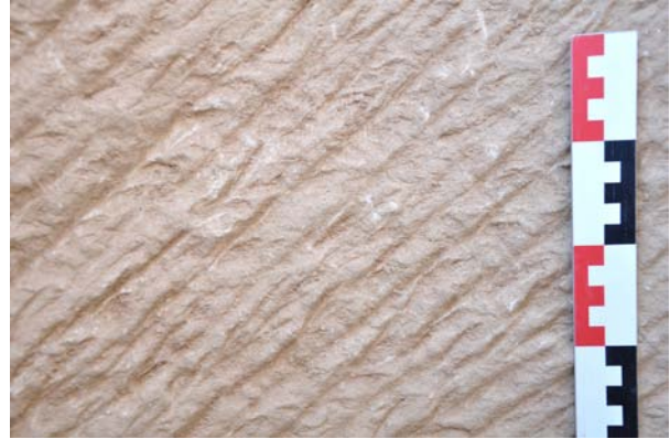
Fig. 64. Inside wall of basin no. 2
