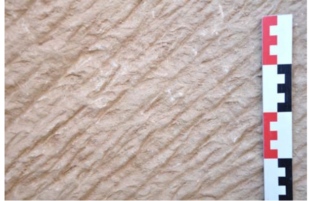
Fig. 64. Inside wall of basin no. 2
