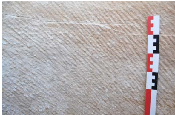
Fig. 61. Bottom of basin no. 1
