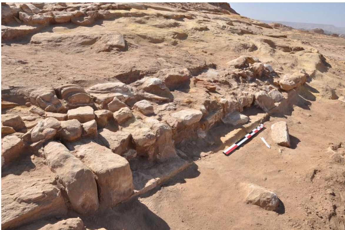
Fig. 77. External terrace wall, from the north. On the right, the blocks rest directly on the bedrock
