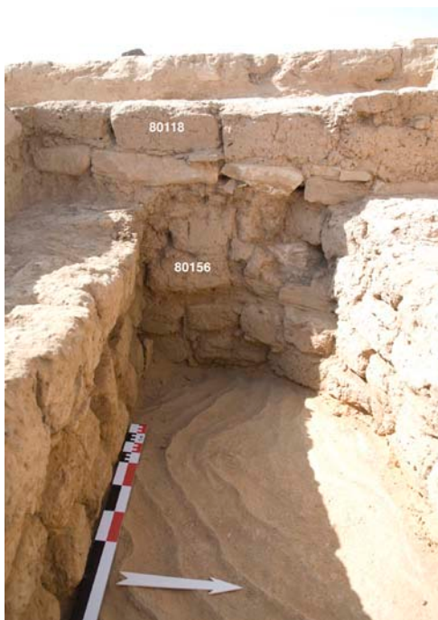
Fig. 10. Sounding F, looking to the west, wall 80157 abuts wall 80156 (center) which turns to the east. Wall 80118 is laid on top of 80156
