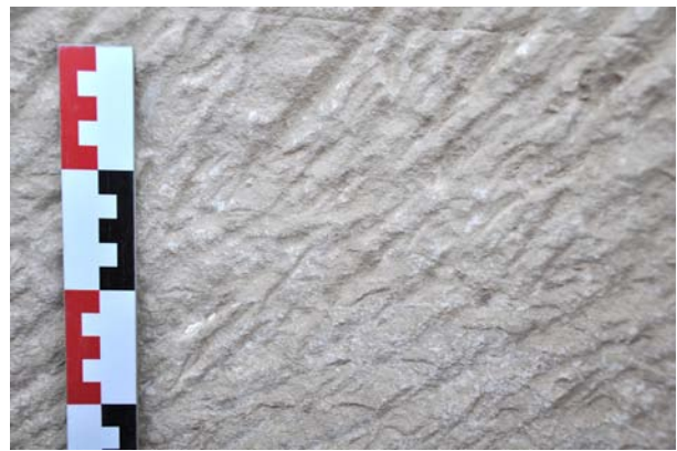
Fig. 66. Inside wall of basin no. 3
