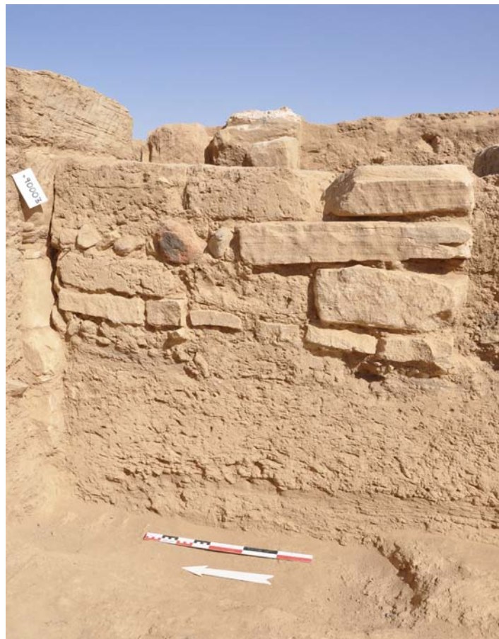
Fig. 11. Wall 90028, from the southwest. In the extreme left is the corner section of wall 90030
