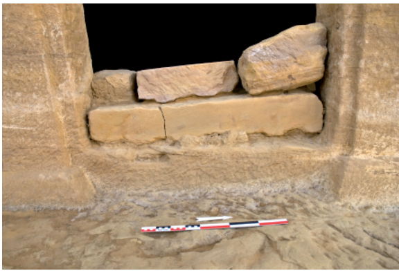
Fig. 28 Preserved courses of the second system of closing the doorway
