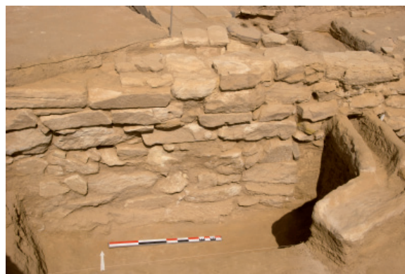
Fig. 13. Wall 20002W – foundation courses and the superstructure. Channel 20014 to the right. View from the south
