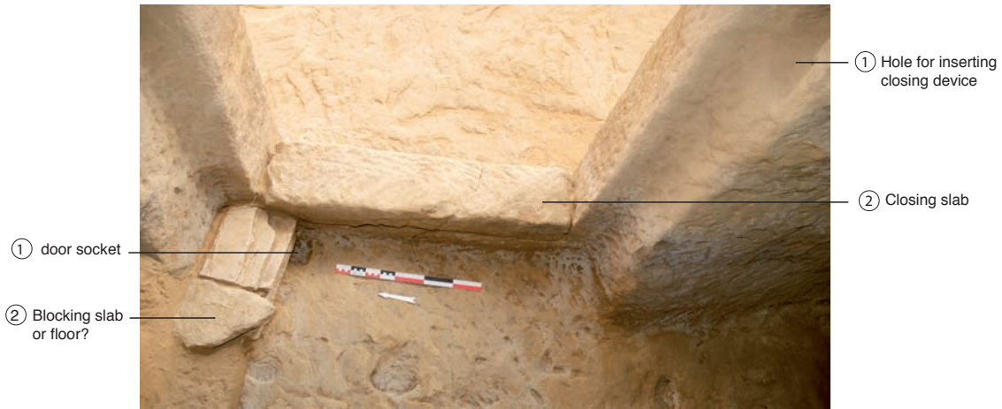
① Element belonging to the first closing system ② Element belonging to the second closing system
