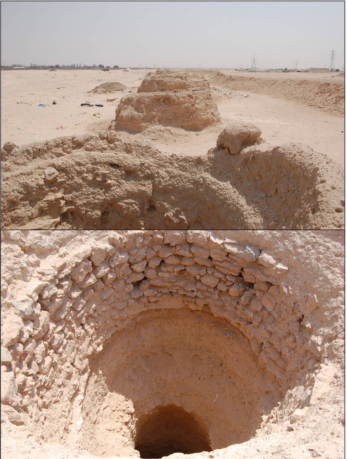
Figure 23: 'Ayn Farzān: wells of the qanat on the ground (top) - inner part of a well (bottom)
