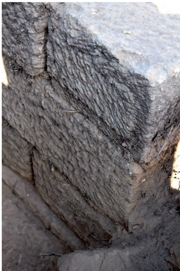
Fig. 14. View of the masonry of the east room. Note the carefully pointed surface and the drafted margin of the upper header.
