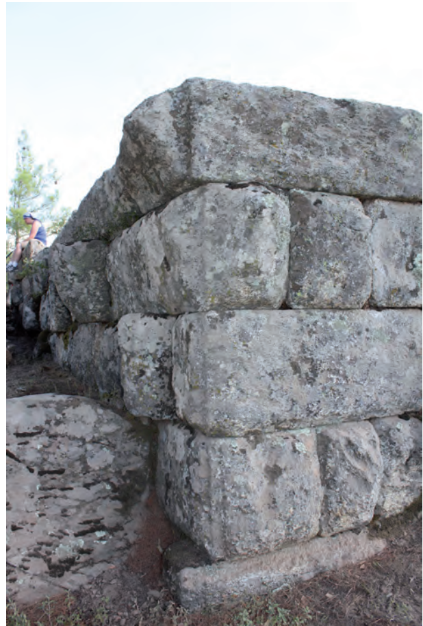
Fig. 7. Double headers at the corners of central tower.
