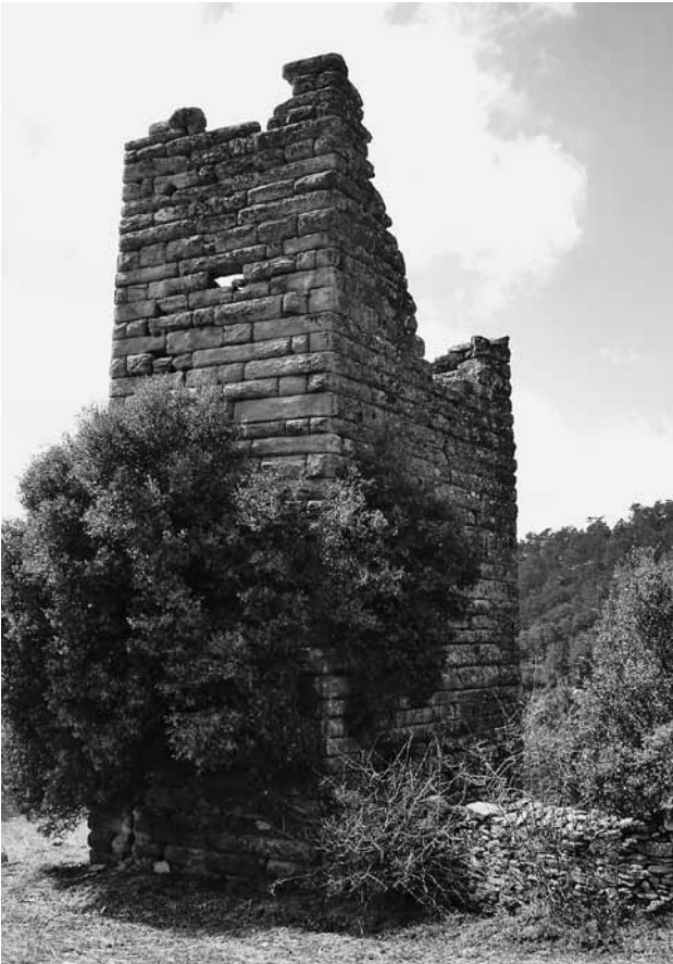
Fig. 4 The tower from the north-east
