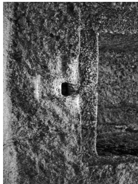
Fig. 18 Swallow-tail shaped cuttings
