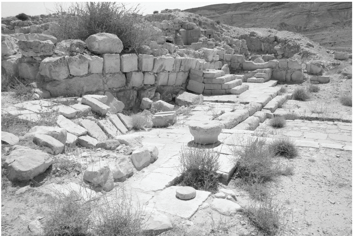
Fig. 6. Façade of room (J) and the upper part of the esplanade (S) deformed by and earthquake (photo P. P.-F. 2007)
