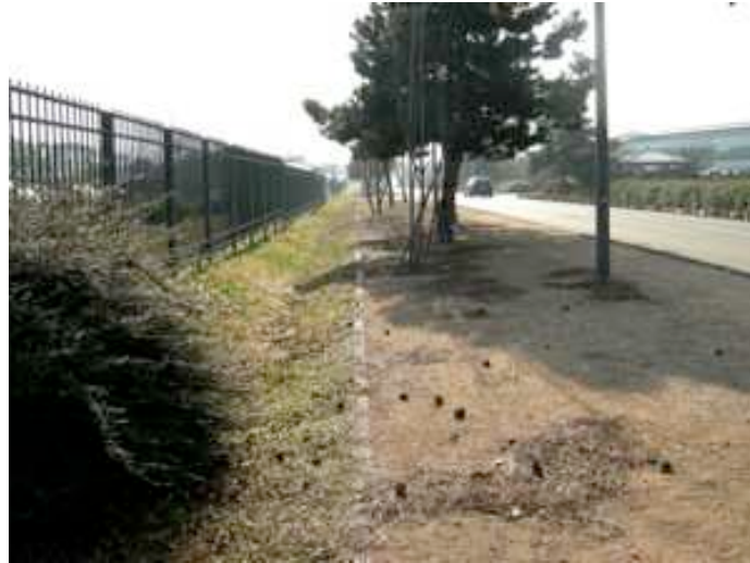
Figure 8. Swale, Irène Joliot-Curie Alley, Technology Park (2011)
