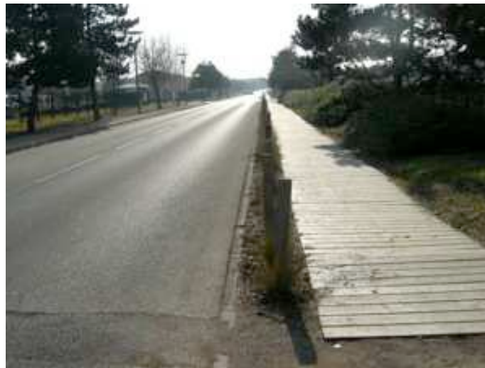
Figure 9. Swale, Irène Joliot-Curie Alley, Technology Park (2011) 2
