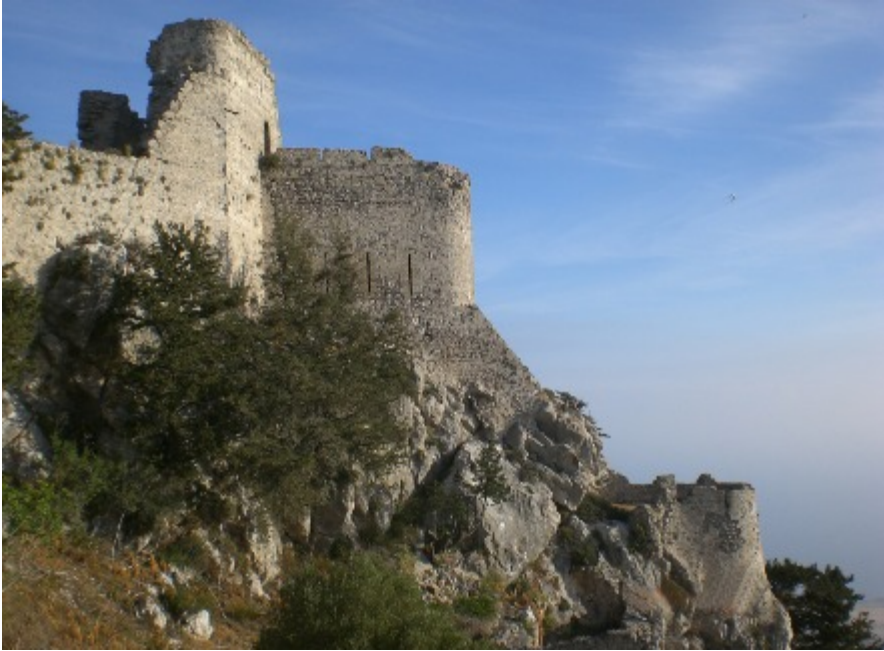
Fig. 11 - The Horse-shoe tower flanking the right-hand side of the entrance to the castle; Cl. Nicolas Morelle, 2008. Defence at two levels is perfectly adapted to the complicated relief features of the terrain. With 7 arrow-loops at each level - one is in the nose - the tower flanks the barbican as well as the platform below it.
