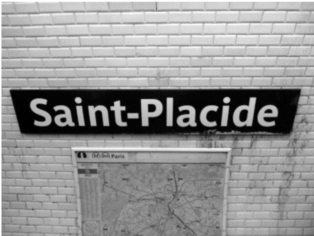
Figure 4. Mold on a signboard
