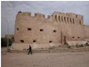
Image 1 – Proto bastion recently (re)plastered. Azemmour 2007 (© R. Carabelli)
