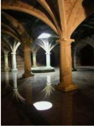
Image 2 – Cistern, interior of the water reserve. El Jadida, 2003 (© R. Carabelli)
