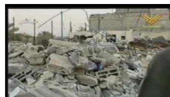
MN11/19 ruined house
