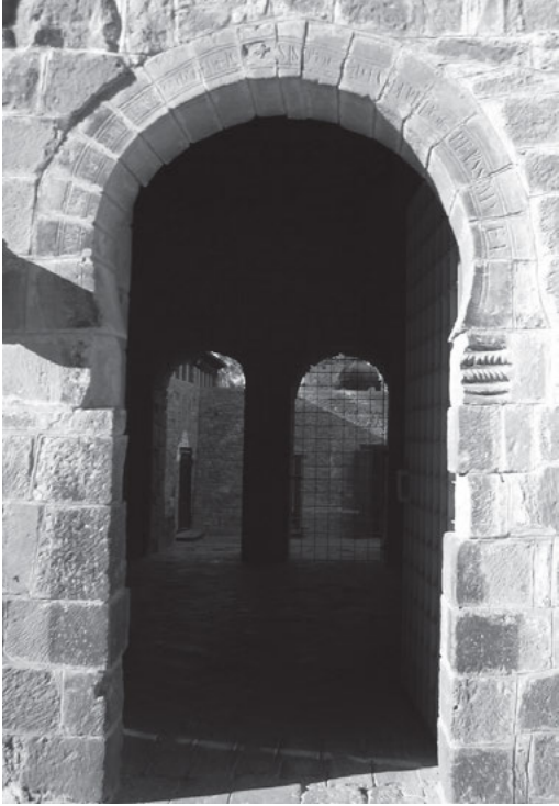
Fig. 3: San Juan de la Peña (Spain), monastery, cloister door © CESC/M/CIFM.
