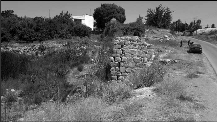
2. Remnants of a late Ottoman water mill at al-Qunayyah (photo Romel Gharib).
