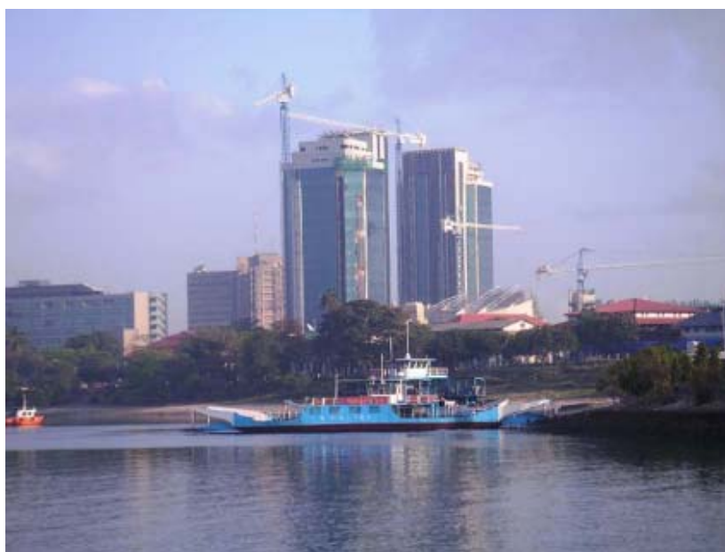
The Central Bank of Tanzania twin towers under construction Dar es Salaam 2005
