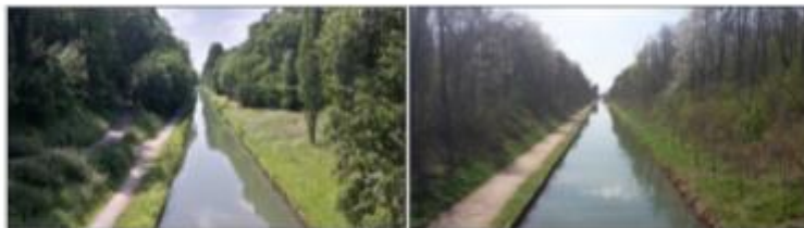
Figure 4 : Two pictures showing the Ourcq channel running below two sloping up berms with vegetation
