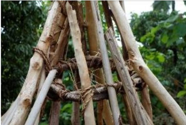
Figure 5: Interior ring *bunkar* on a damaged roof (Orodara region, June 25, 2016)
