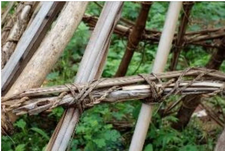
Figure 6: Interlacing *kaar-ja mon* on a damaged roof, Orodara region (June 25, 2016)
