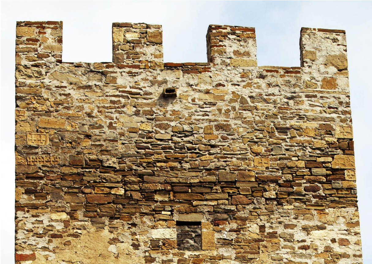
Fig. 17. Sudak (Sugdeïa/Soldaïa, Crimea). Tower of the Genoese consul Federico Astaguera (1386). South façade. Photo A. Dzhanov.
