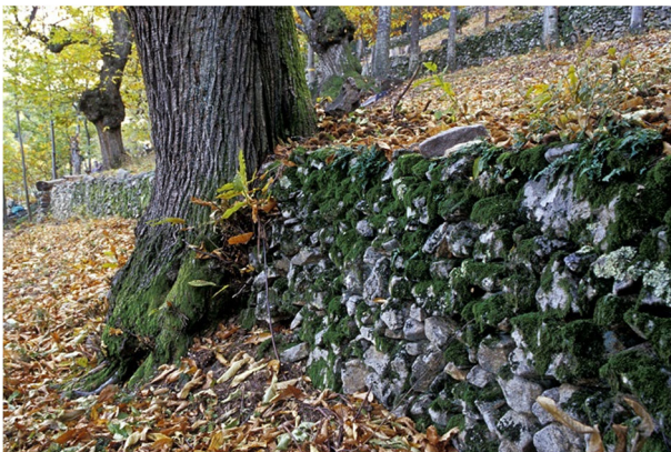
Châtaigniers – Boutières – (photo Cica-Rissoan)
